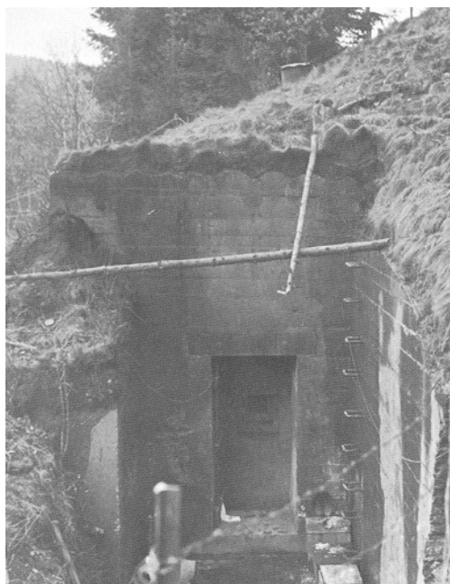
TYPICAL PILLBOX. Above (left) exterior, showing door with firing embrasure. Interior of firing embrasure at right. Below (left) bunk area, and (right) ventilation device.
